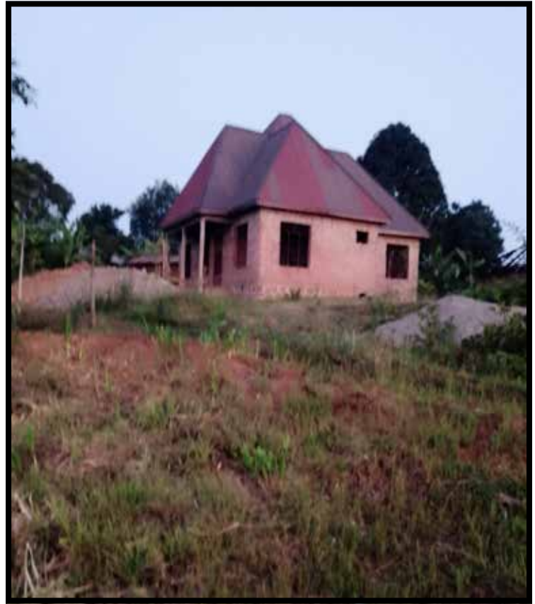
Figure 6. The home currently under construction for Judge Ephraim's parents.
