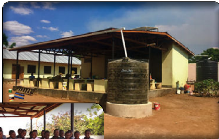
Water tanks fed by rain gutters.
